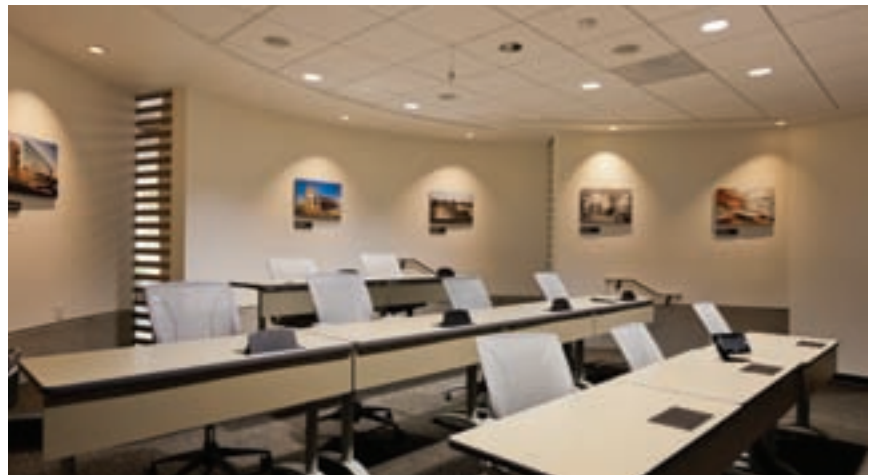
LED downlights were used in this auditorium, as well as hallways.
