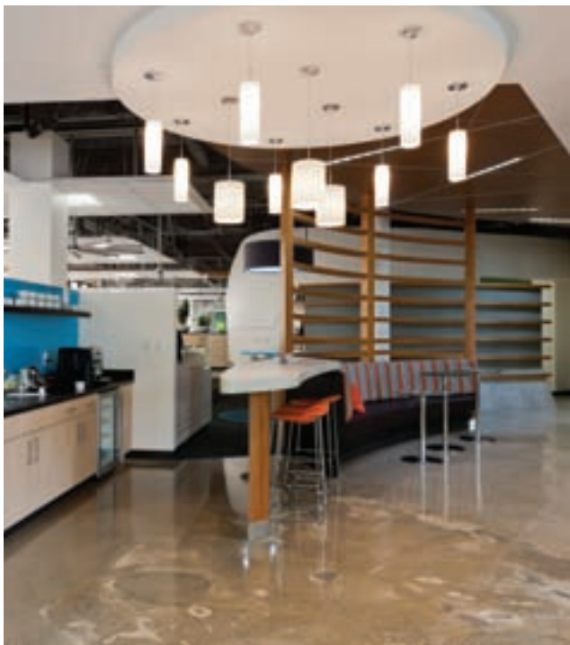
Pendant lights in the kitchen are part of the all-LED system.
