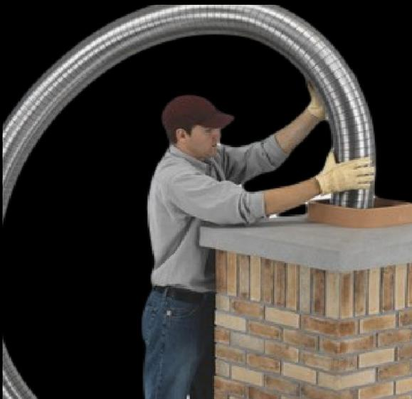
Once installed, a chimney liner would need regular inspection to check for undesired creosote and soot build-ups, cracks, leaks or any other kind of damage it may have.
