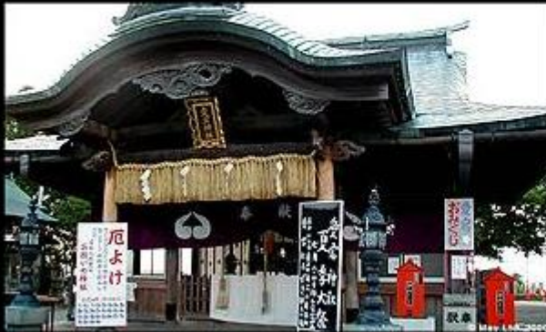
• Main shrine building ⇨
