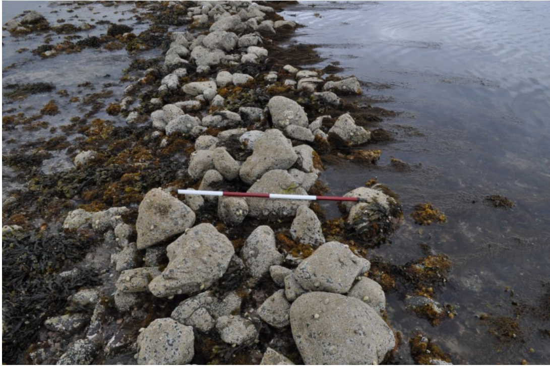
Looking down on the wall near the centre.
