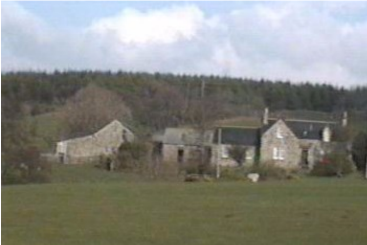
Kilfinan farmhouse and outbuildings - much the same as they were after being renovated during the trusteeship
