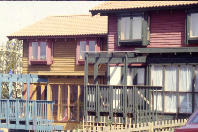
Early days Diggers self build
