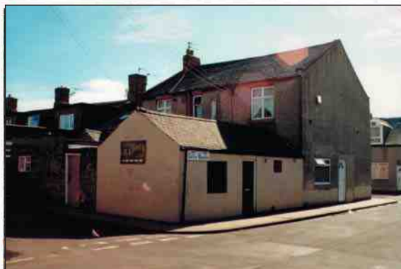
58 Castlereagh Street (2002) showing barber's shop in foreground
