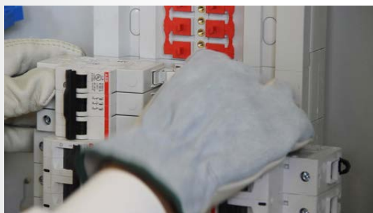
The Breaker Snaps Into The DIN Rail
