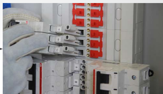
The Breaker Is Inserted Into The Opening
