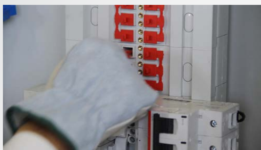
The Protective Cover Is Removed
