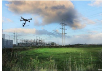
Power Line Inspection
