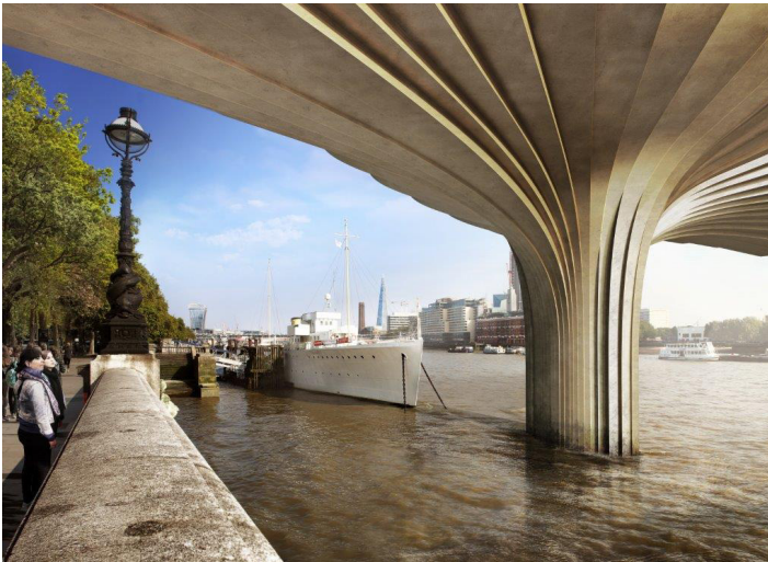
SLIDE IR 8 © ARUP North Bank – Victoria Embankment showing close position of the north 'planter' to embankment
