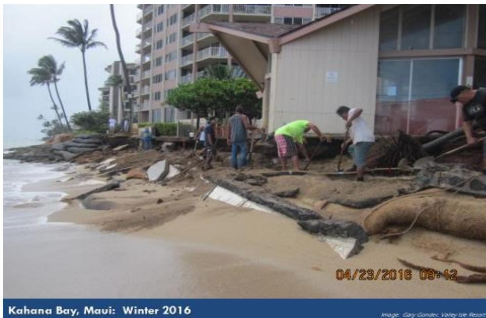
**Figure 2. Damage to sand bags, pool deck, and uninhabited cabana at Royal Kahana AOA, April 2016.** Valley Isle Resort suffered similar beach erosion. All shoreline parcels are at risk due to continued erosion as well as failure of existing seawalls.
