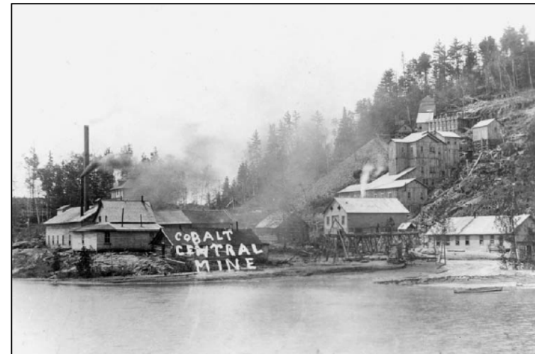
Source: Geological Survey of Canada report
