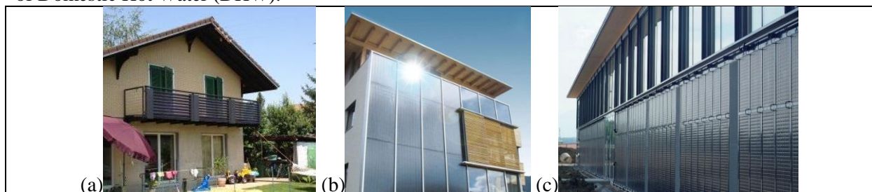
Figure 2: Integration solutions of (a) vacuum tube [3], (b) flat plate [4] and (c) unglazed technologies [5]
