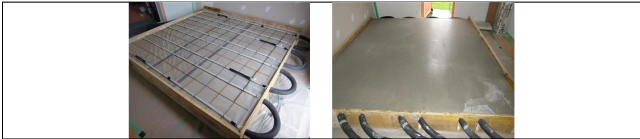
Figure 7: Test on prefabricated slabs [10] in the Kubik by Tecnalia test facility.
