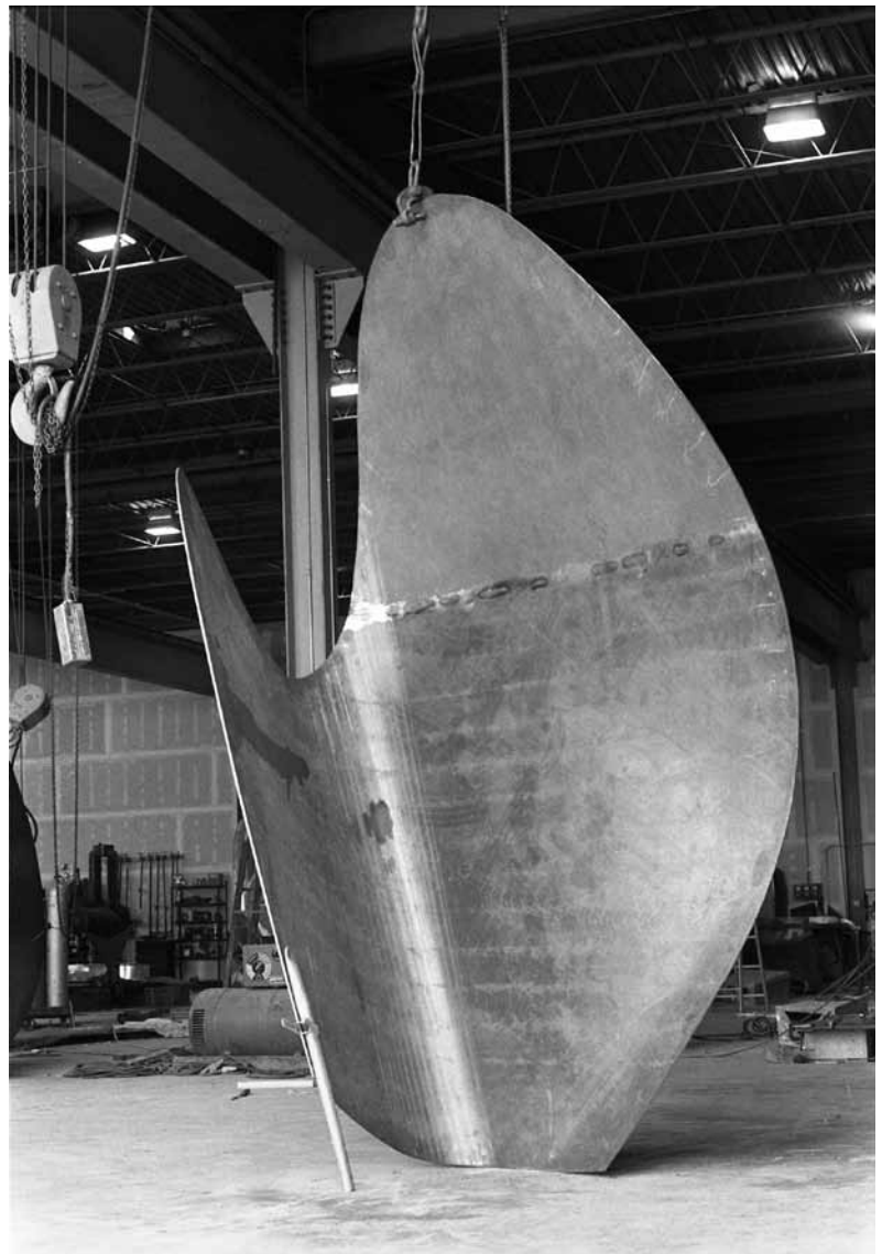
The steel shell of Mitt , placed upright for study and to determine the method of support and the base structure.
