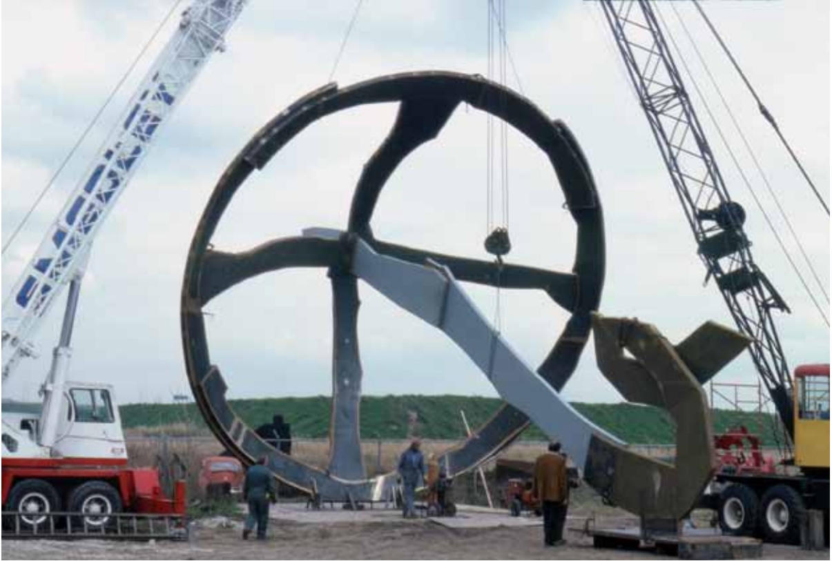
Crusoe Umbrella during the initial test assembly, prior to the finishing work
