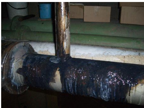
Applying pipe wrap Seal PLUSresin & activator
