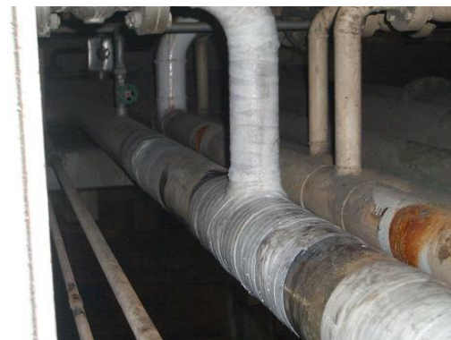
Applying Wrap Seal™ fiberglass tapes
